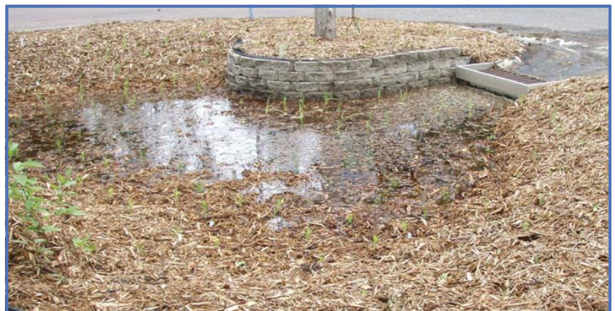
Curb-cut rain garden location and corresponding drainage area.
