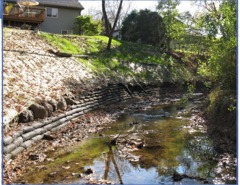
Completed project early in the fall of 2011.
